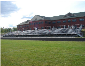
Workers put the finishing touches on the permanent bleachers.
